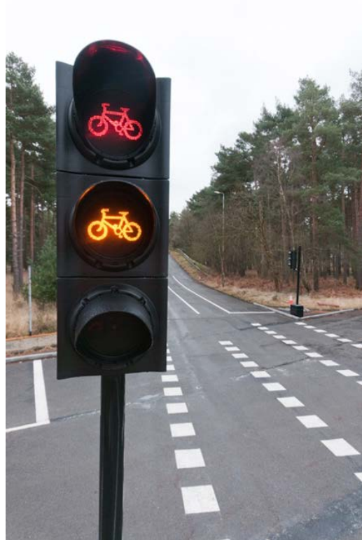
Figure 4 – Trial signal heads (Cycle Red)
